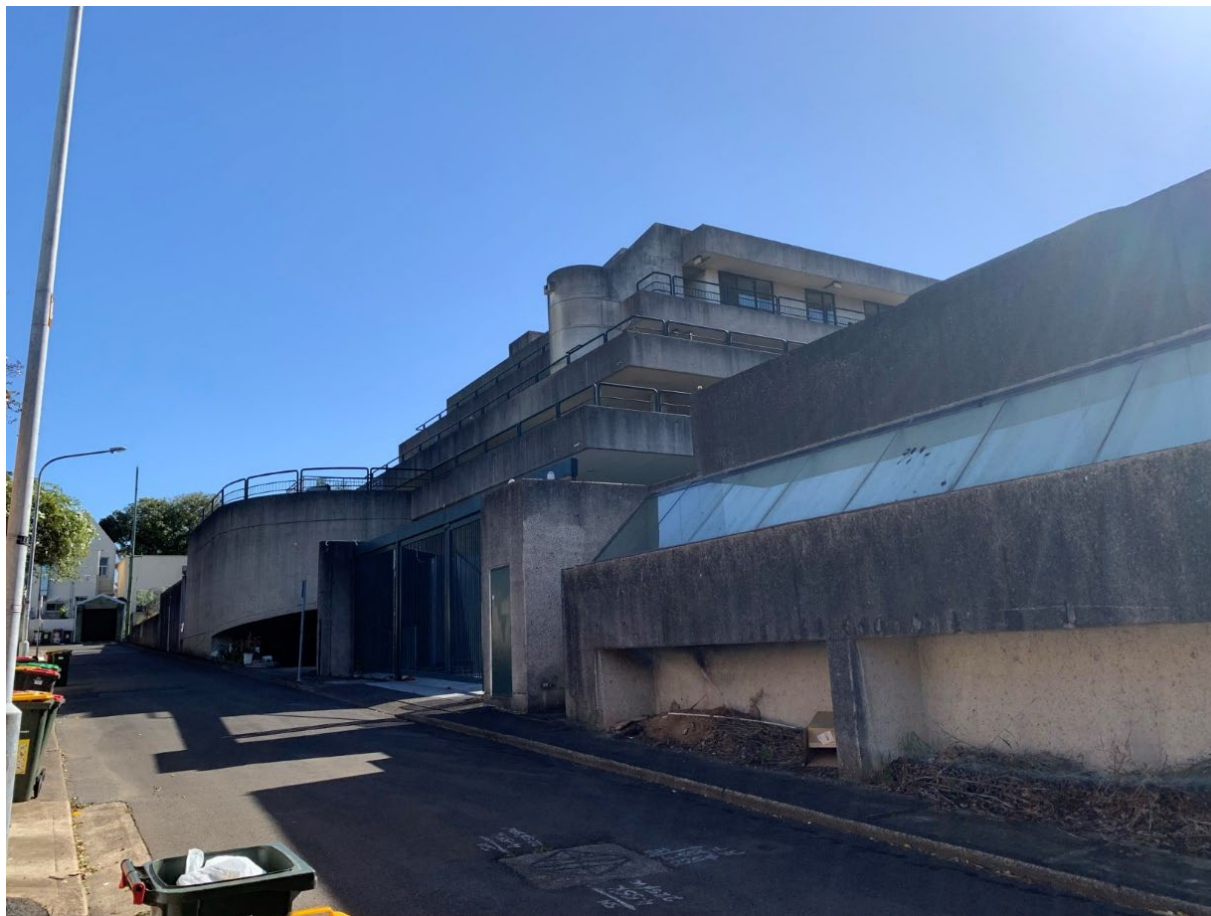
Ferry Lane elevation of MRC Building (south)
